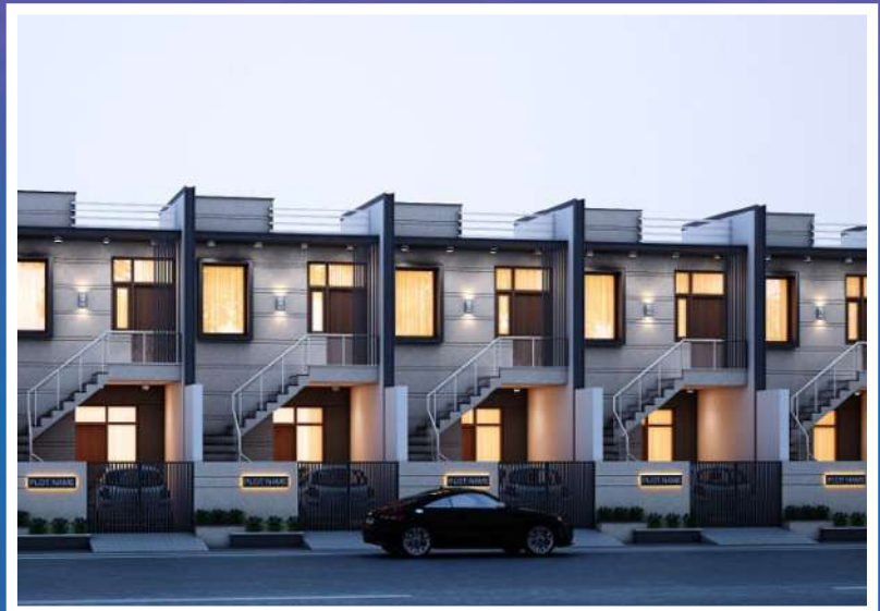
VINAYAK RESIDENCY Sirsi Road, Bindayaka, Jaipur Row Houses on the developing outskirts of Jaipur.
